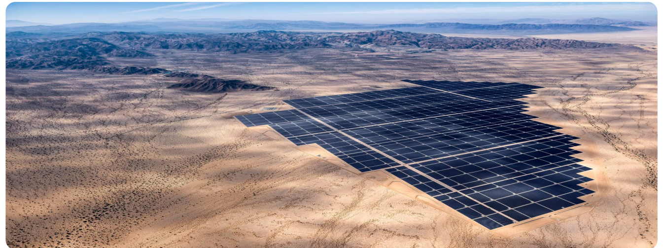
550MW Desert Sunlight Solar Farm (source: TIME)
